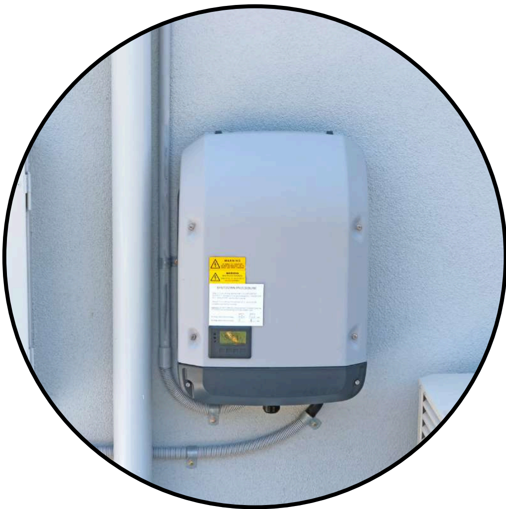
Inverter Wiring for Individual Flat
