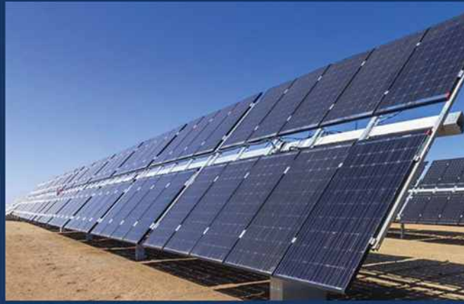
SOLAR SYSTEM FOR LIFT & COMMON AREA
